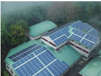
Dewalakande roof top solar project
